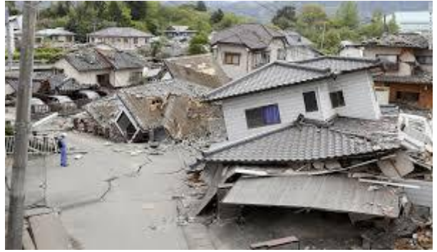
Fig 4: Houses along earth's line of weakness
