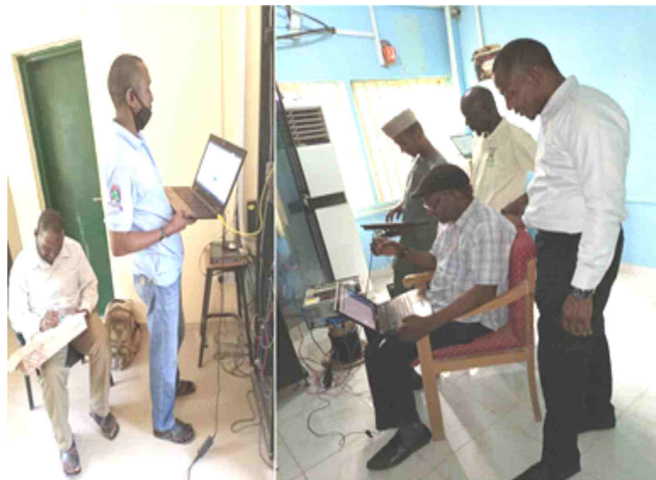
Members of Network Administration Unit in Data Centre and Server Room
