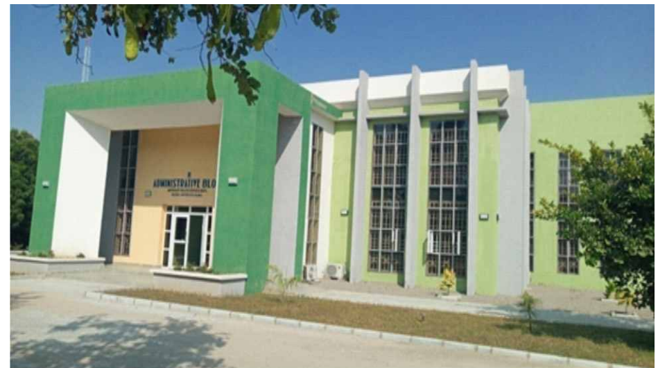
The Administrative Block
