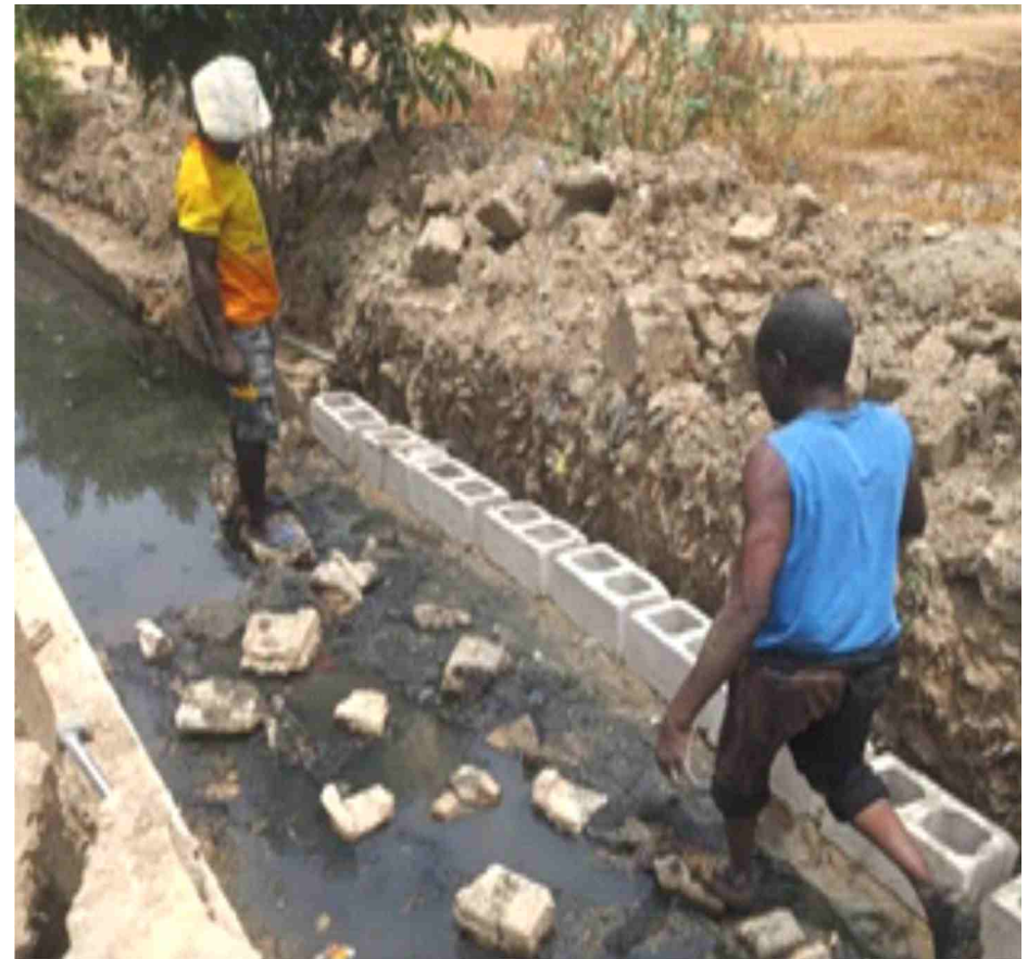
Reconstruction work of collapsed wall at SCE
