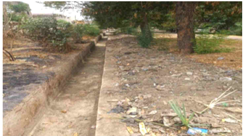
Drainage desalting and reconstruction of collapsed wall section
