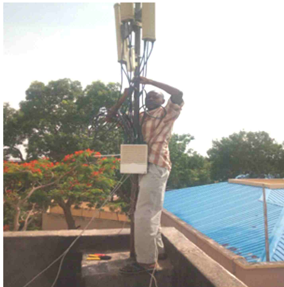
A NAU member performing restoration of a Wireless Access at the ASUU Secretariat
