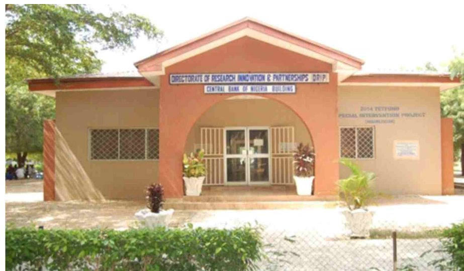
Front view of the Directorate of Research, Innovation and Partnership (Intellectual Property and Technology Transfer Office)
