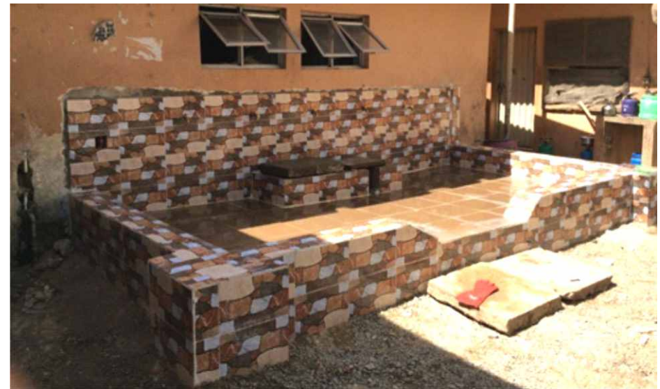
New open laundry at Block E, Nana Hall
