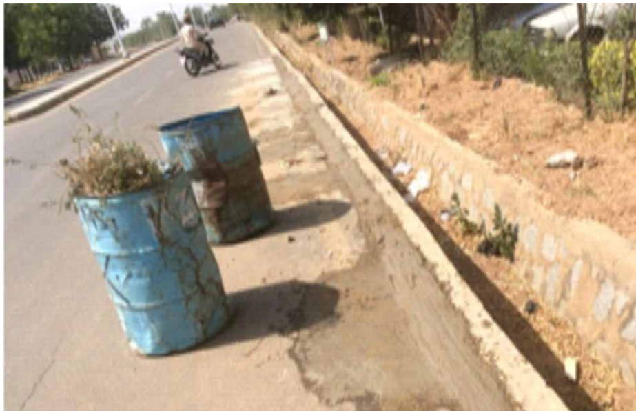
Some of the constructed drainages
