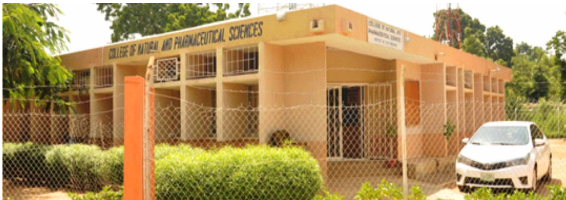
Provost office complex
