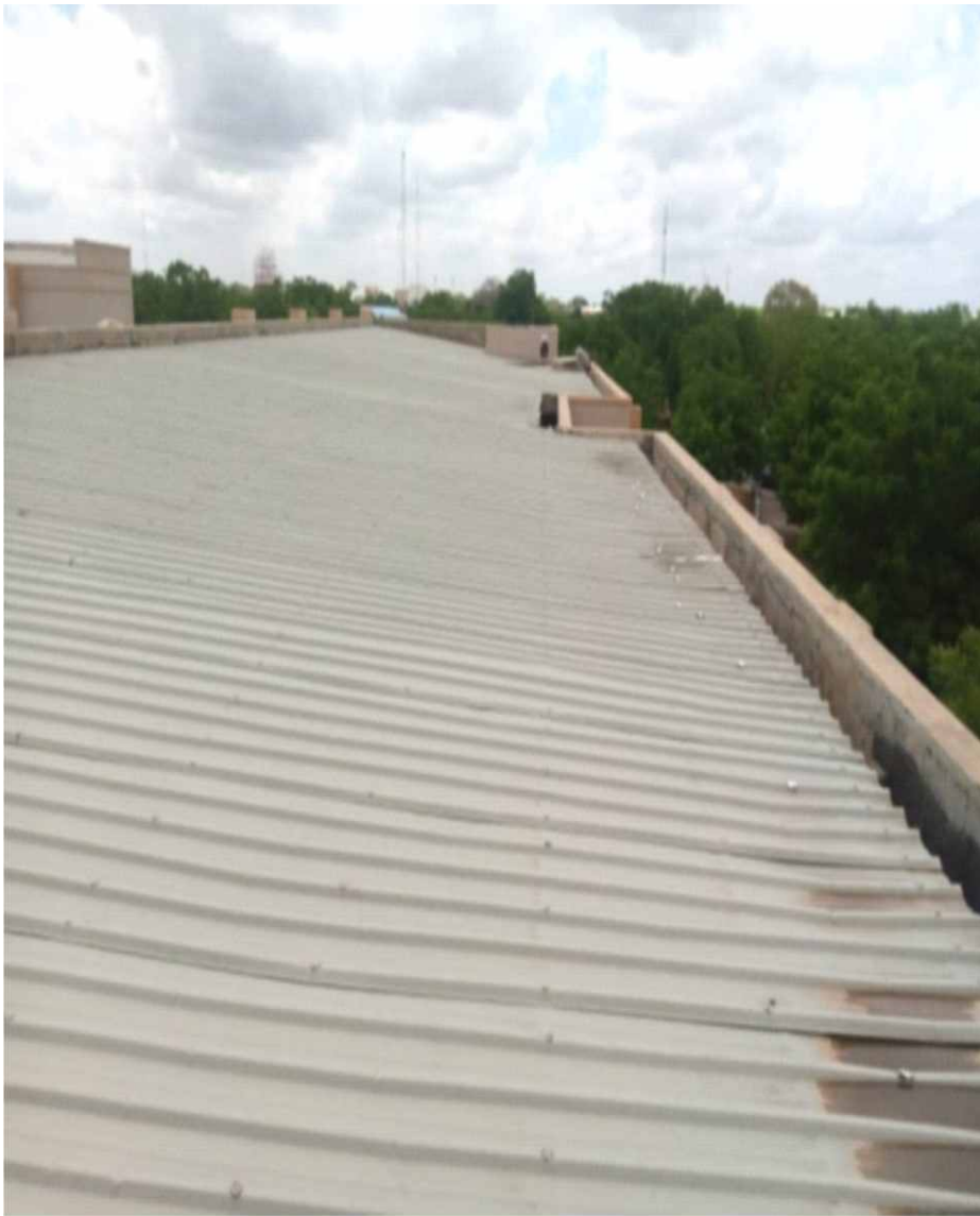
Renovated Faculty of Law Roof
