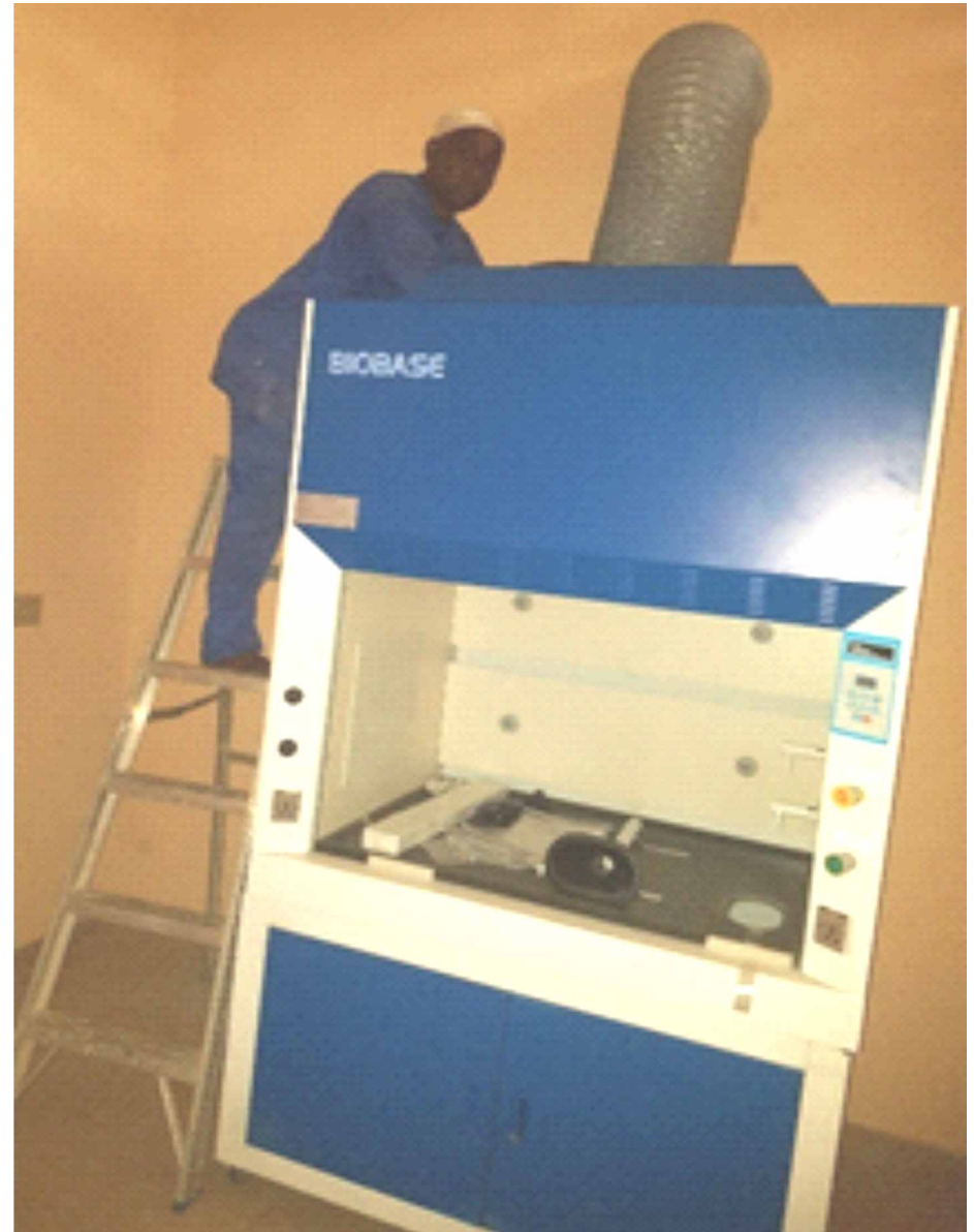
Fume Hood Installation
