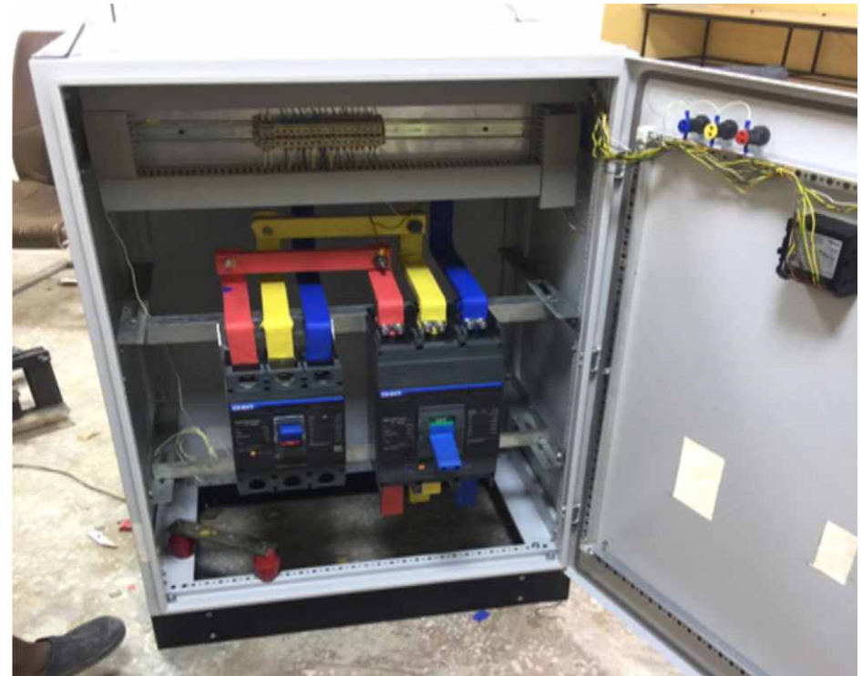
Installation of change over switch for the student hostels at the new campus
