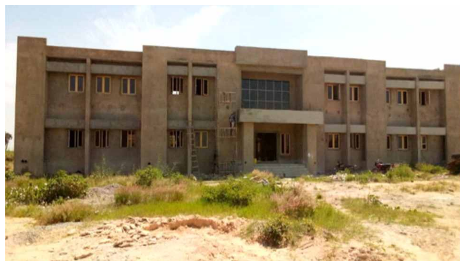
Department of Veterinary Anatomy (Under Construction)
