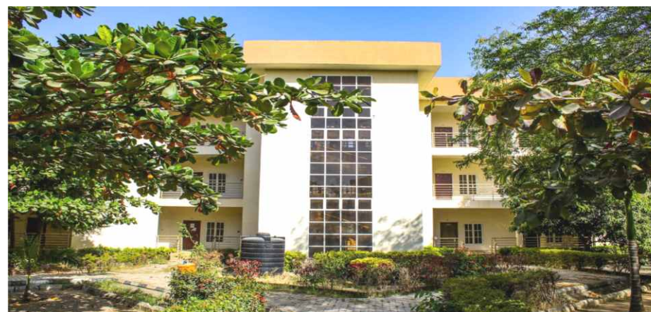
Inner View of the Faculty Building
